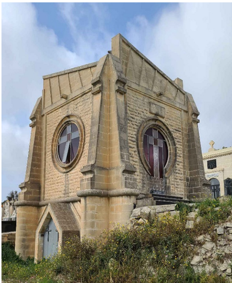
Figure 8: Chapel built over small bluff. Photo courtesy of John Odell.
